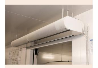
The refrigeration cell has 3 air curtains at the doors, model ACA-E-B-S, type B including circulation of ambient air. The air curtains are installed just above the doors in the refrigeration cell.
