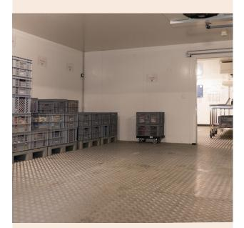
The floor is enforced with a load distribution plate. The floor panel has a wooden insert of 15 mm and an aluminum chequer plate.
